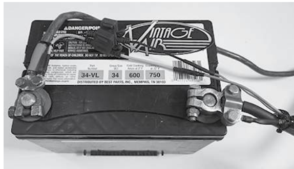
Completed Installation Shown
