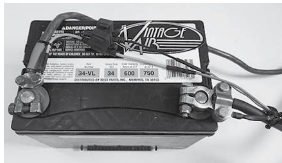
Completed Installation Shown
