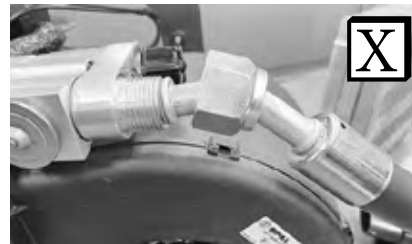
Improperly Seated O-ring Land
